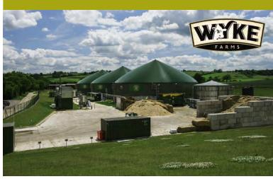
Anaerobic digester plant producing power to make cheese at Wyke Farms
