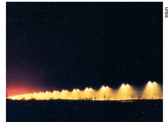
Full Cut Off lighting illuminate the road without lighting up the night sky
